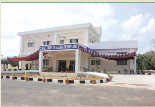
2MIGD Reverse Osmosis Desalination Plant
