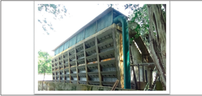
Figure 4 Revamped Main Cooling Tower
