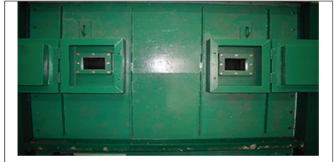
Figure 5 Viewing window of SG casing
