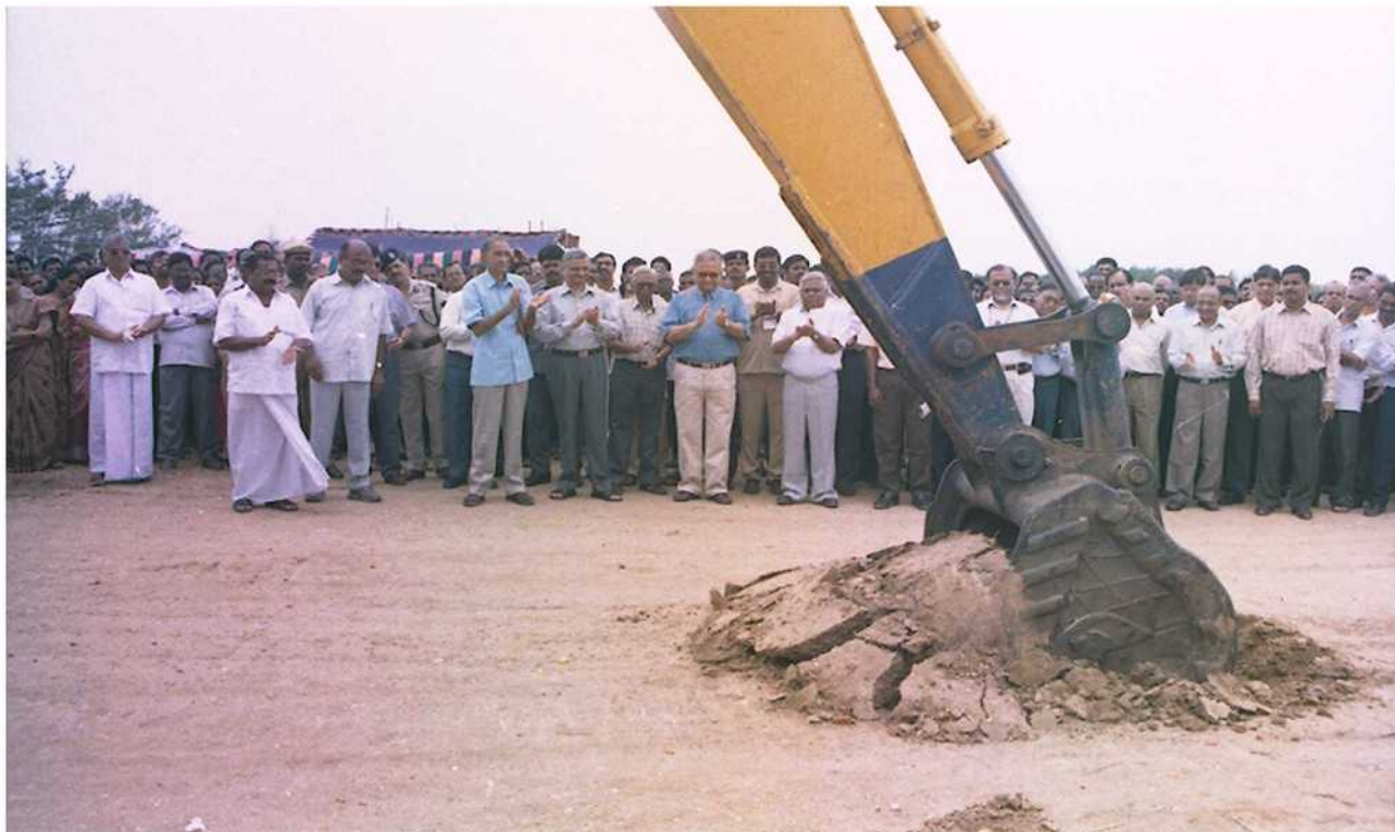
Ground breaking function for the commencement of excavation work on Nuclear island of PFBR on 18 th August 2003. Dr. Anil Kakodkar, Chairman, AEC & Secretary, DAE, Dr. B. Bhattacharjee, Director, BARC, Shri S.B. Bhoje, Director, IGCAR and Heads of other DAE units participated in the function.
