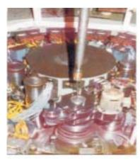
Fig.2 In-situ Cutting of Guide Tube on the Reactor used in 1988
