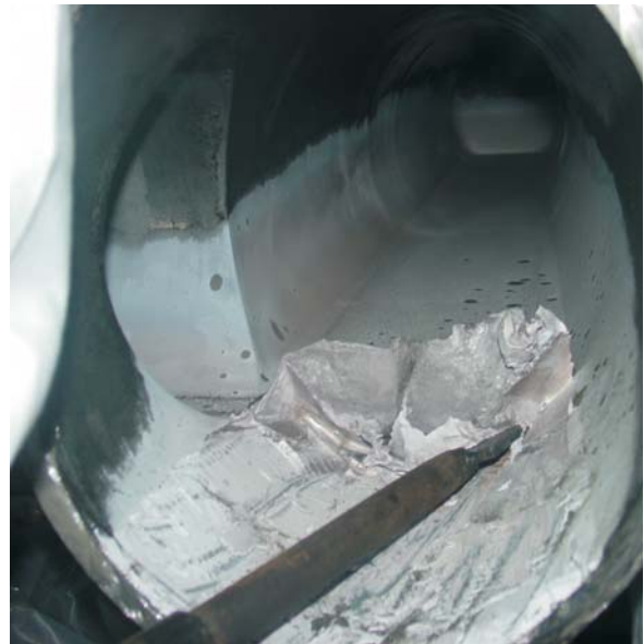
Figure 3 : Frozen sodium after removing the SG rupture disc
