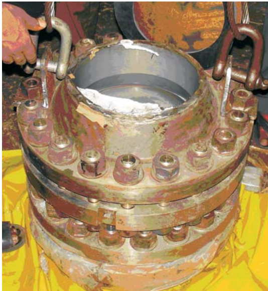
Figure 2 : Removed steam generator rupture disc assembly
