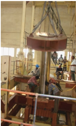
Figure 3: Primary ramp with primary ramp liner
