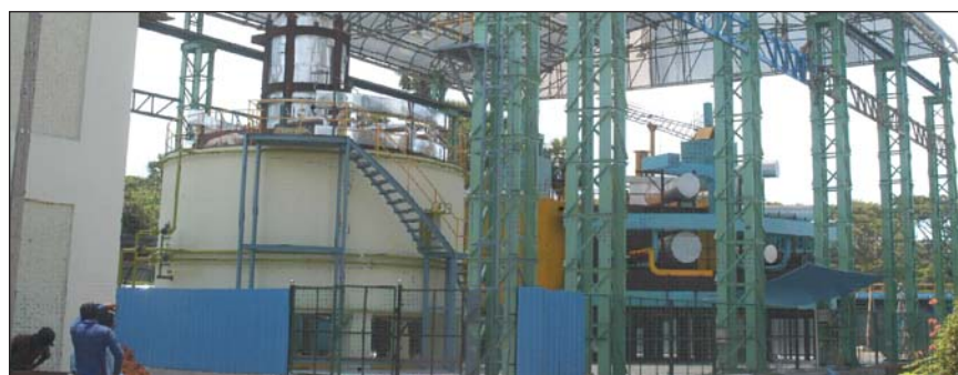
Fig. 2 Overall view of facility
