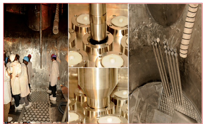
Fig. 3 Erection of outer B 4 C subassemblies
