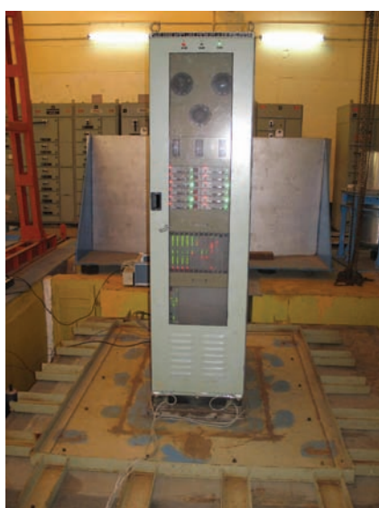
Fig. 1 PCSL system at shake table
