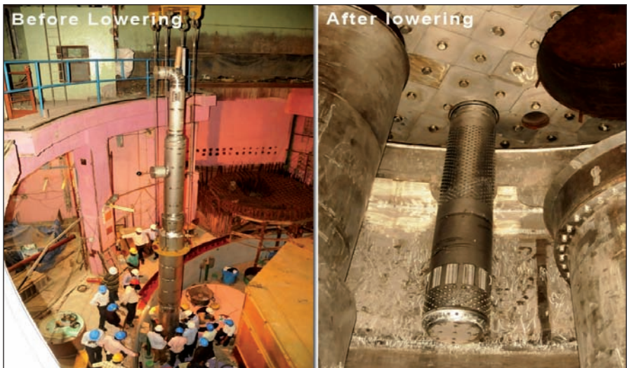
Fig. 1 Erection of decay heat exchangers through roof slab penetration
