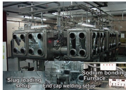
Fig. 1 Argon atmosphere negative pressure glove box train with various facilities
