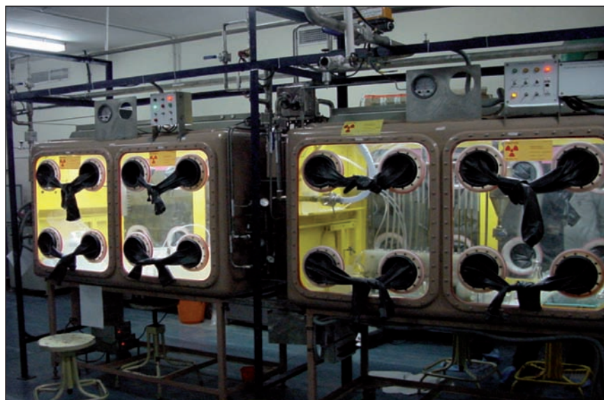
Fig. 1 Mixer-settler facility for flow sheet development studies
