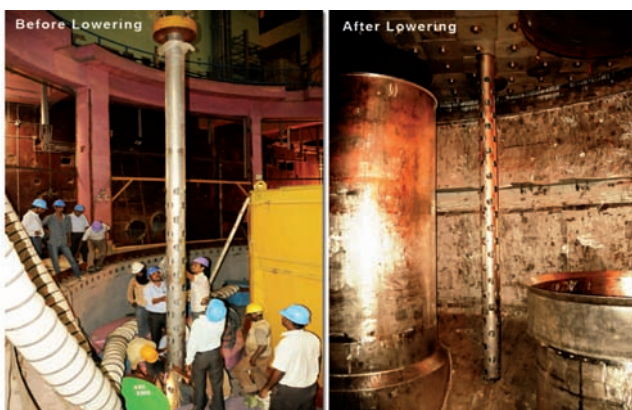
Fig. 2 Erection of hot pool level detector inside inner vessel
