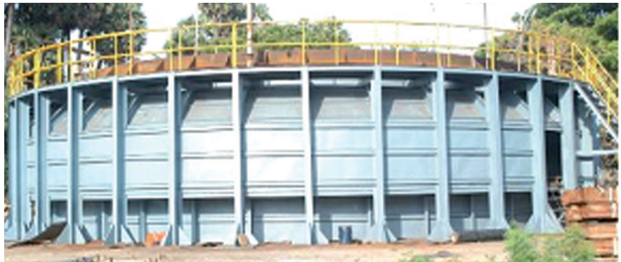
Fig. 3 Mockup trials for the successful erection of safety vessel
