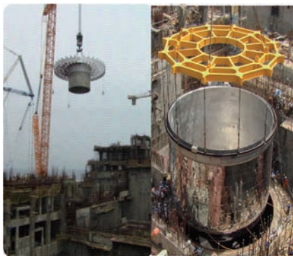
Fig. 4 Mockup trials for the successful erection of safety vessel
