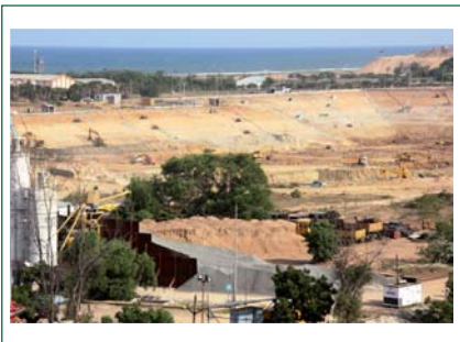
Fig. 1 Excavation in the nuclear island area for construction of plant buildings
