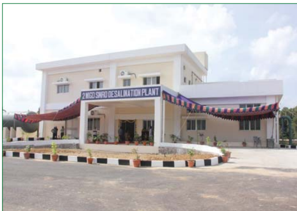
2 MIGD Reverse Osmosis Desalination Plant
