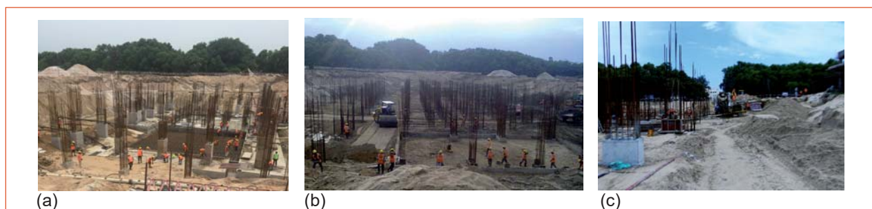
Fig. 1 Photographs of STC construction site
