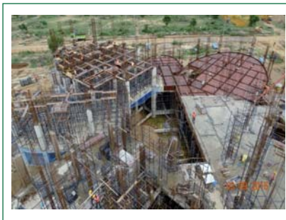
Fig. 2 Training Centre of FRFCF under construction
