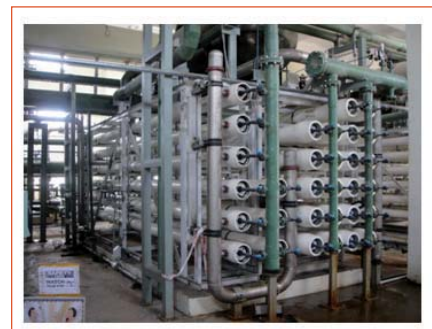
Fig. 3 Reverse osmosis membrane skids to remove the dissolved salts
