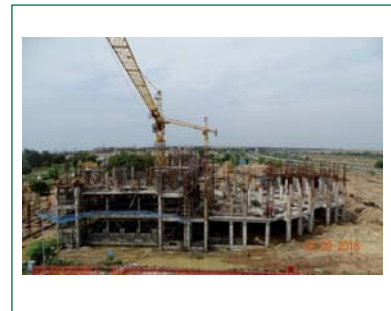
Fig. 3 Administration building of FRFCF under construction
