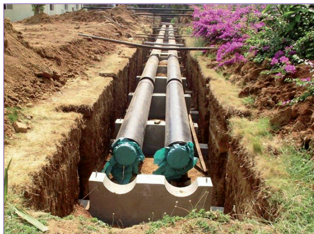
Fig. 2 Erection of pre-insulated underground pipes
