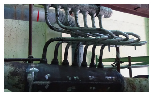
Fig. 3 Header with thermal baffles welded in-situ
