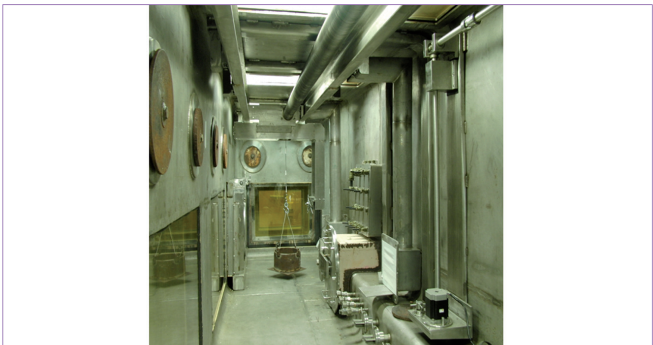
Fig. 2 A view of in-cell crane inside lead cell containment box
