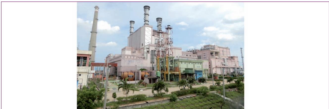
Fig. 1 West side view of PFBR
