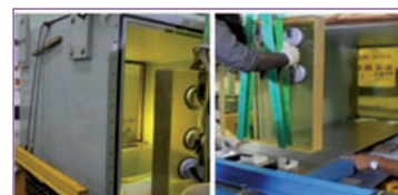
Fig. 6 Window glass removal using vacuum cups
