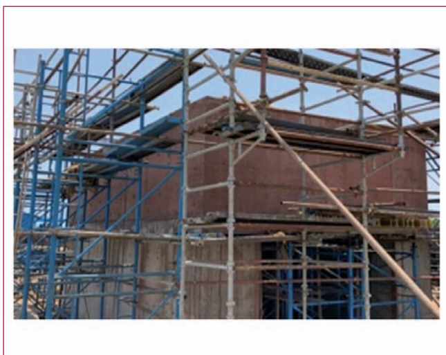
Fig. 1 Full scale mockup slab
