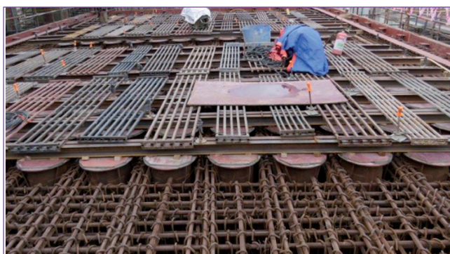
Fig. 1 View of pin vault prior to concreting
