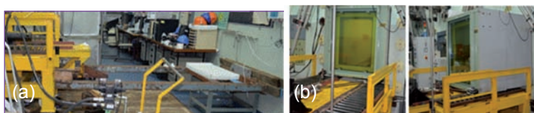
Fig. 4 (a) Structural support structure mounted with the trolley and (b) RSW retrieval from the liner brick wall
