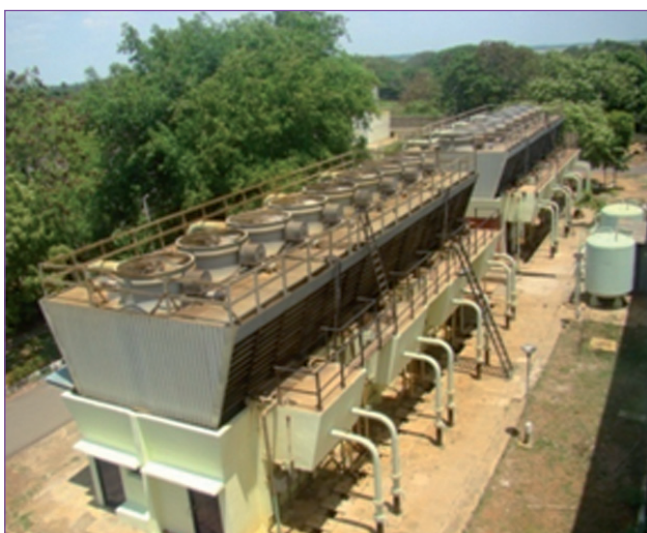
Fig. 1 CWCP cooling tower after revamping
