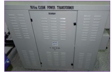
Fig. 3 50 kVA Dry Type isolation transformer
