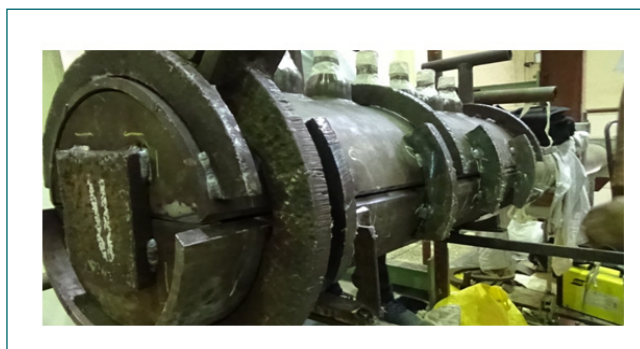
Fig. 2 Inlet header long seam and circular joint fit up
