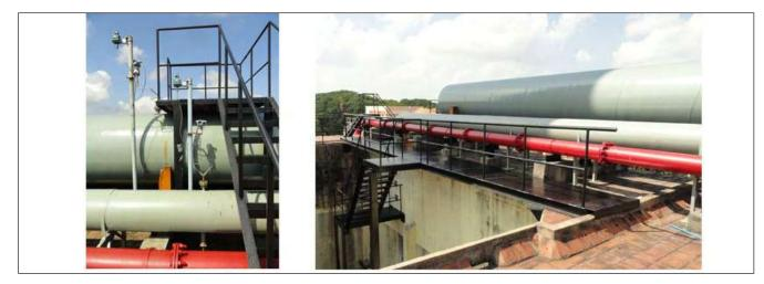
Fig.1: APT in the plant exhaust duct along with wireless adapter fitted on DP transmitter
