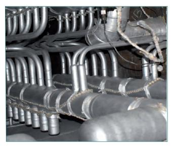
Fig. 2 Tubes of SG after normalisation
