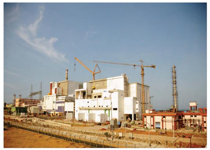
Fig. 1 Overall view of turbine and nuclear island connected building
