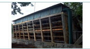
Fig. 1 FBTR 50 MWt cooling tower before revamping
