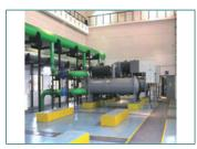
Fig. 1 CWCP-II high-bay with chillers and associated piping network
