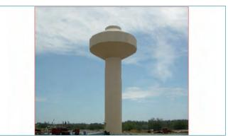
Fig. 12 Picture of completed Intze Tank
