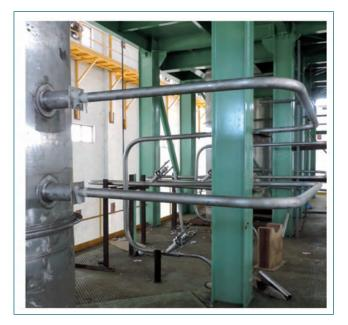
Fig. 1 Overflow and outlet pipe lines
