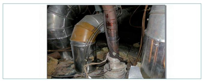
Fig. 1 Hot argon line (insulation removed) in B4 cell
